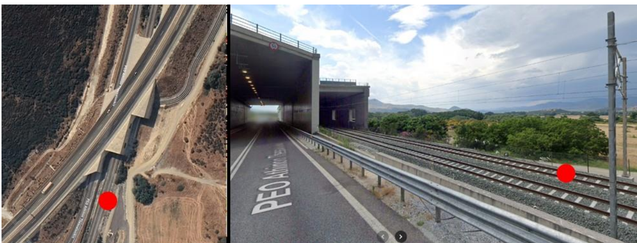
Figure 3. Photos of the tunnels on the site of the accident (left, satellite – right, from the road beside)
