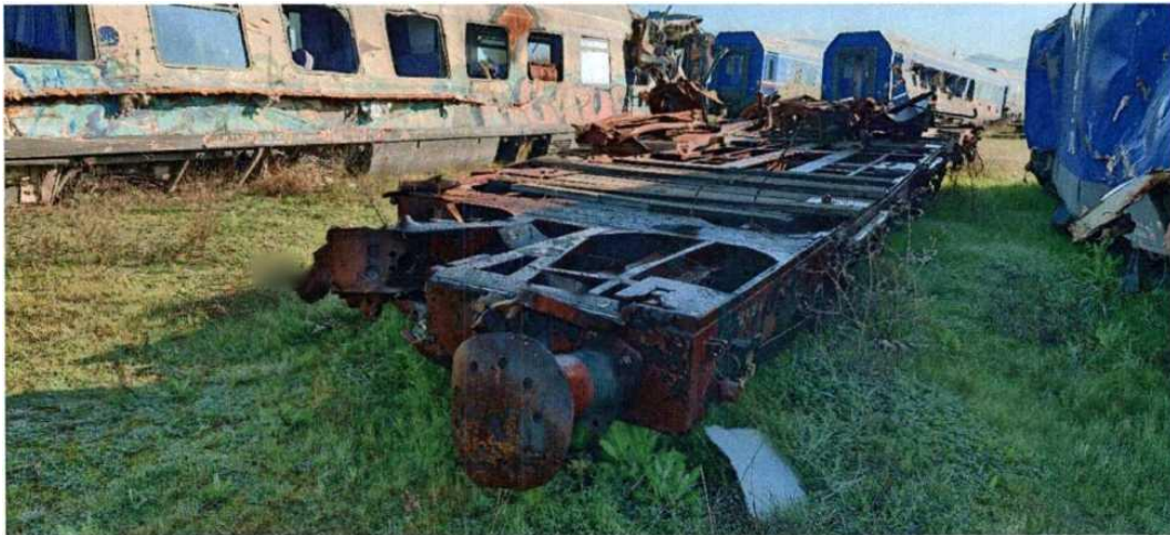
Figure 79. Position 3) nr 1 platform carrying steel plates, front half totally destroyed by heavy impact with Restaurant Car.
